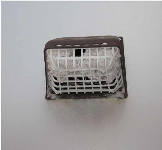
Figure 4. Note the potentially dangerous lint build up on this screened dryer vent.
